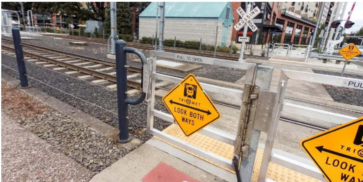
Figure 3.14: Passive gates close off both sides of the crossing closets to the light rail
