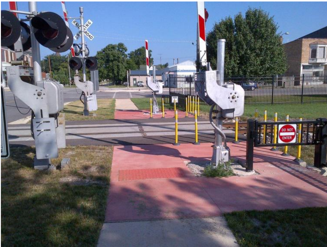
Figure 5.9: Pedestrian Automatic Gates (N/A, N/A, n.d.)
