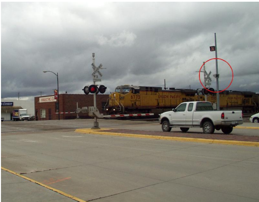
Figure 5.4: Wayside Horn System (APWA Reporter, 2007)
