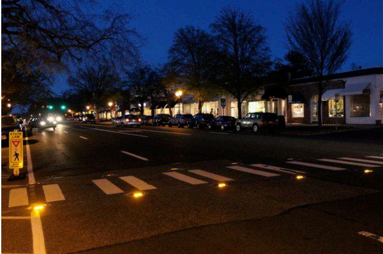
Figure 5.5: In-Pavement Marker System (Bromley, 2013)
