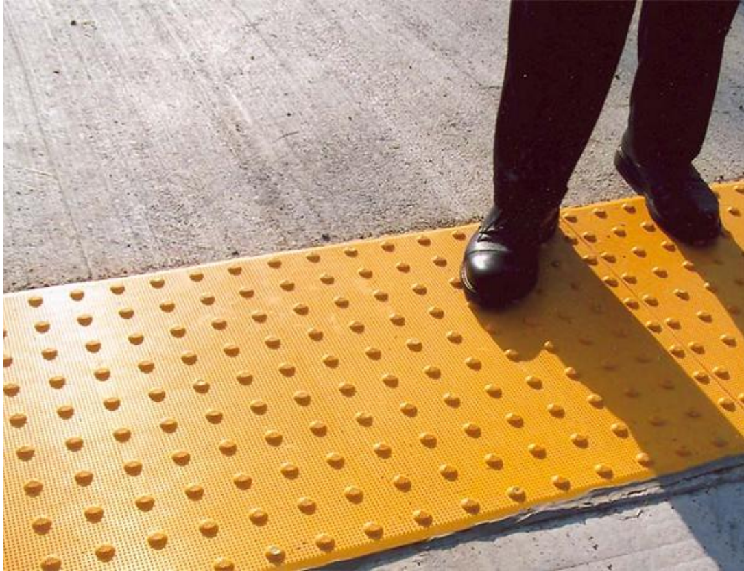
Figure 5.17: Tactile Warning (N/A, N/A, N/A)
