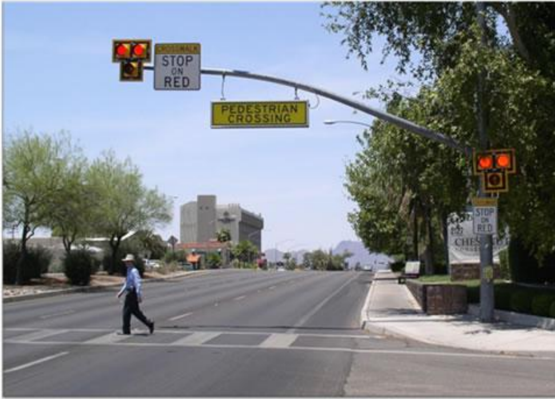
Figure 5.10: High-Intensity Activated Crosswalk (HAWK) (USDOT FHWA, 2016)
