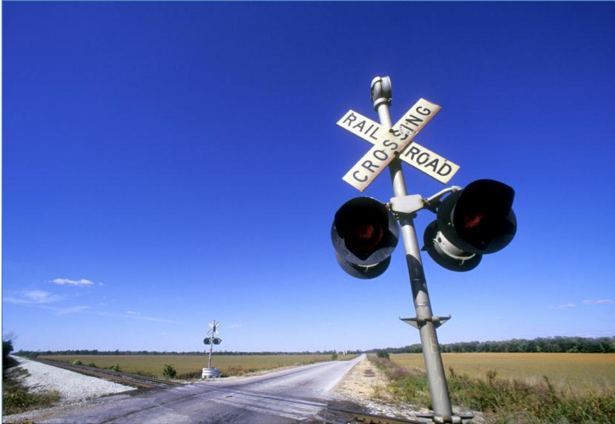
Figure 5.1: Flashing Light Signal (Mixon, 2015)
